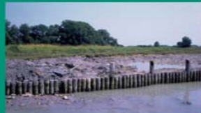
Wooden piles (test edge)
